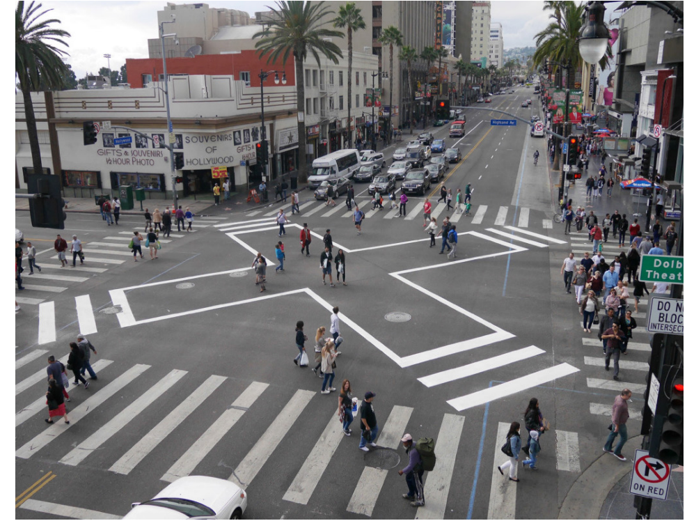
Diagonal crossing marked with paint
