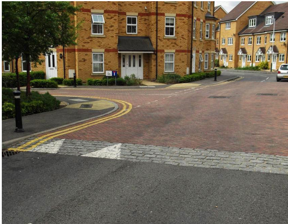
Raised intersection with material change
